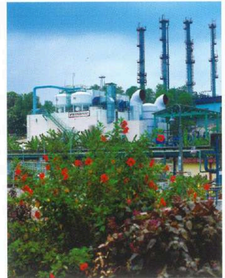
Oxygen plant at BPCL Refinery
