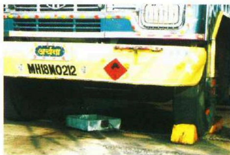
Tray arrangement provided under a tank lorry to check spillage at Manmad Installation
