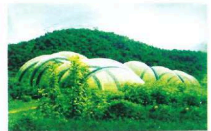
A view of the Butterfly Park at Numaligarh refinery
