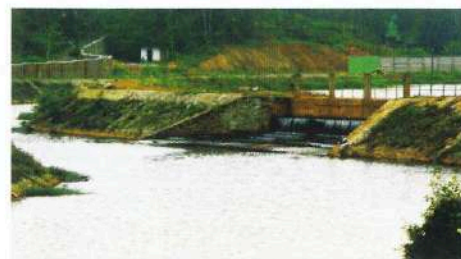
Rain water harvesting at Kochi refinery
